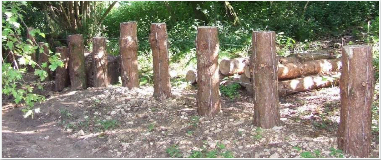
Figure 1. Example of stumps reinforced to prevent winching and chainsawing (Scenario E above)
