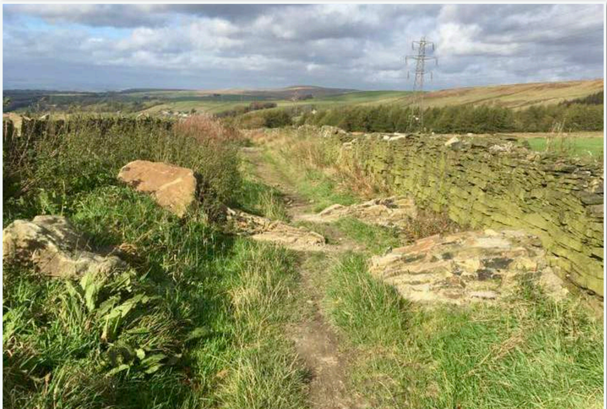
Figure 2. Example of 'cross axle humps' or 'axle twistors' to prevent conventional cars and vans from accessing this green road, which helps to prevent fly tipping and the dumping and/or torching of joy-riden cars, without preventing recreational use (Scenario J above).
